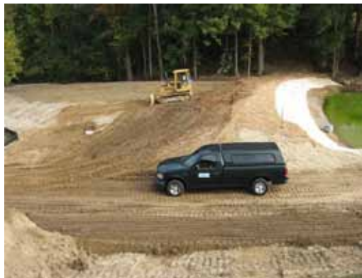
Dam and Outlet Repair
