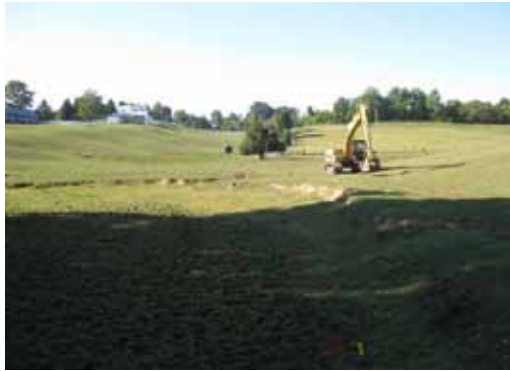
Repair Work on Pond (Before)
