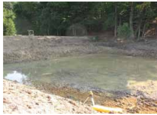
Excavation Repair Work
