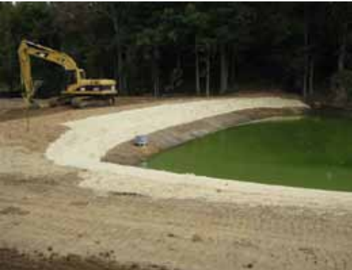
Dam Work Grading and Seeding
