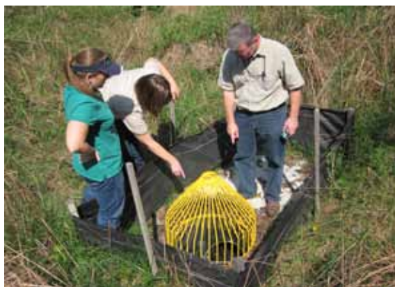
Inspecting the surface inlet of a recently completed Grade Stabilization Structure.
