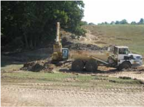
Excavation for Cattle Ramp
