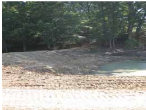
Dam and Principal Spillway Repair
