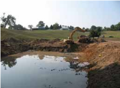
Excavation Repair Work for Cattle Ramp
