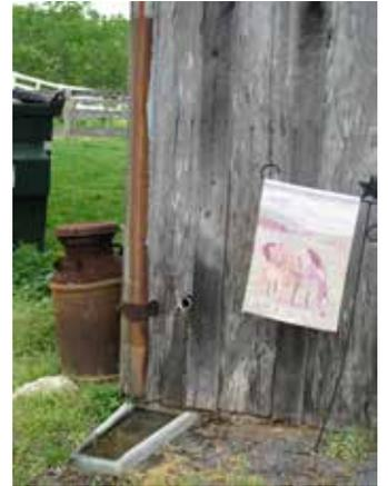
Erosion washed away the soil around portions of the foundation, permitting water to flow into the barn. Attempts were made to keep stalls and storage areas dry. Plywood, flexible tubing, and stone dust had been brought in to raise the elevation of the stalls. Yet water still pooled in the barn, soaking the soil under stall mats, creating nutrient and potential animal health problems.
